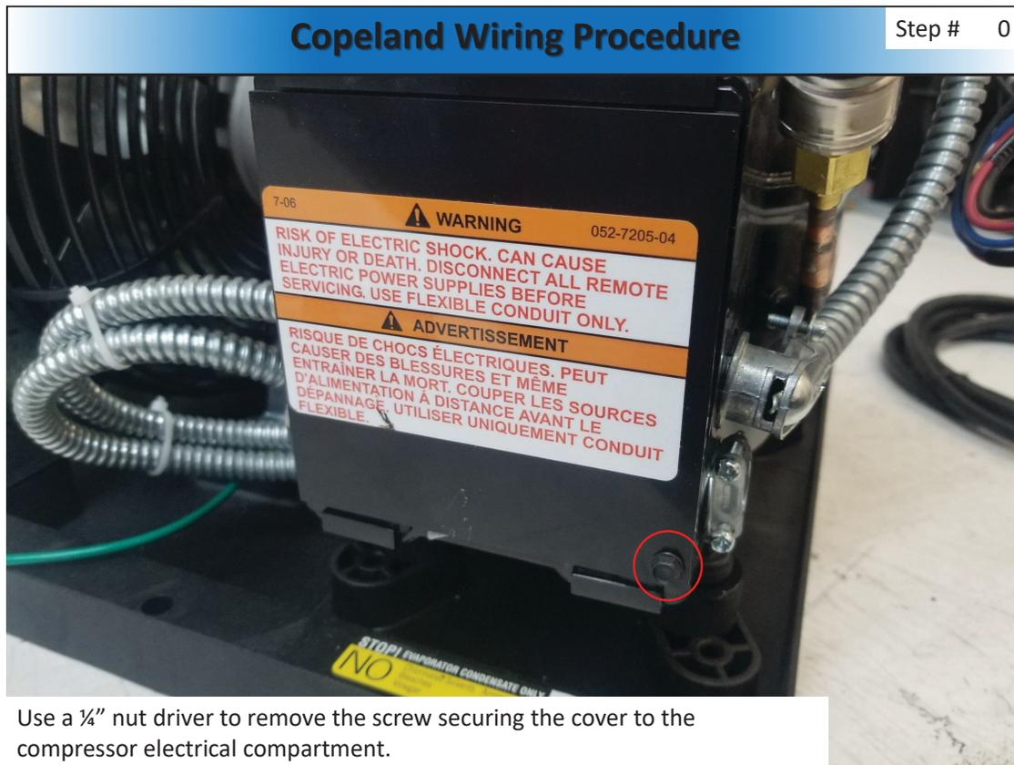
Use a ¼" nut driver to remove the screw securing the cover to the compressor electrical compartment.
