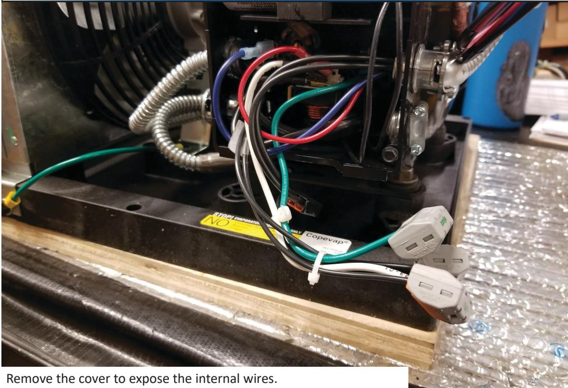
Remove the cover to expose the internal wires.
